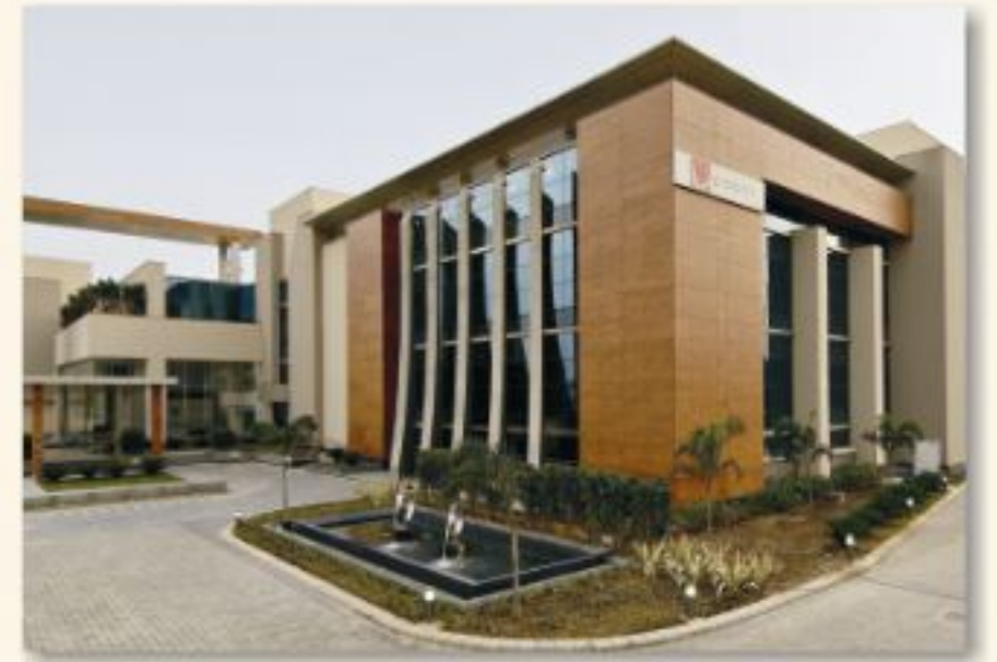
PATNI KNOWLEDGE CENTRE, NOIDA (BLOCK A) PLATINUM RATED LEED CERTIFIED GREEN BUILDING - 2008
