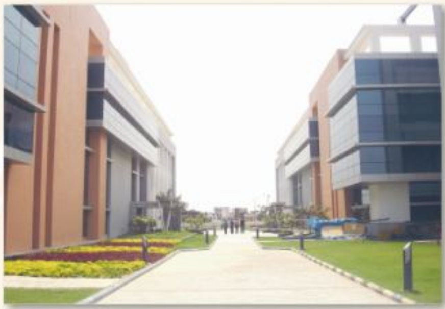
WIPRO TECHNOLOGIES, GREATER NOIDA GOLD RATED LEED CERTIFIED GREEN BUILDING - 2009
